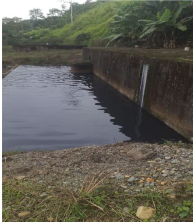
Figure 6. Diagnosis of the sludge drying bed
